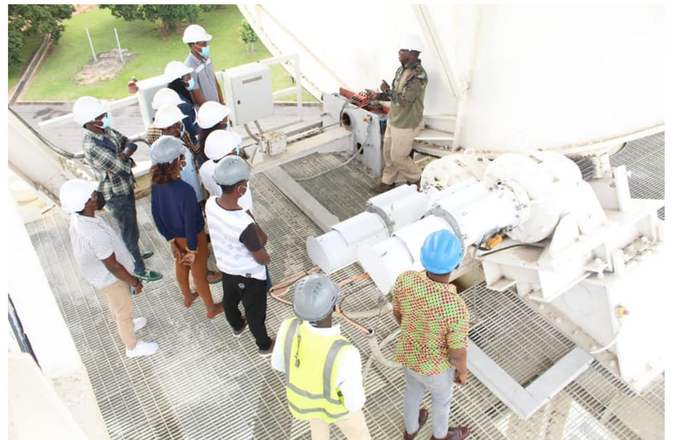
Figure 3: Training on various components of the 32-meter dish
